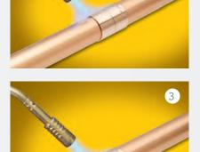
**3.** Apply solder to the mouth of the fitting. When the correct temperature has been reached the solder will flow freely and be drawn into the joint. Briefly reapply the blowtorch and wipe off any excess solder.
