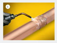
**5.** Apply the filler rod to the mouth of the fitting, allowing the brazing alloy to melt and flow into the annular gap.
